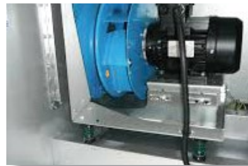
Plenum fans help reduce noise levels
